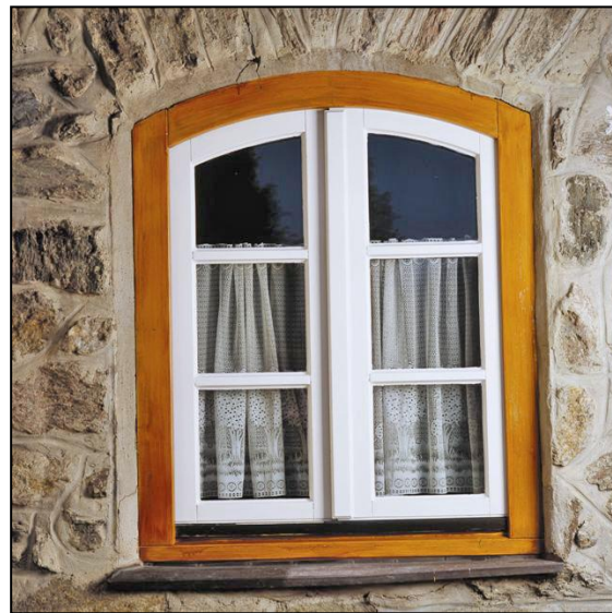
Fig. 4.3: After renovation coating
