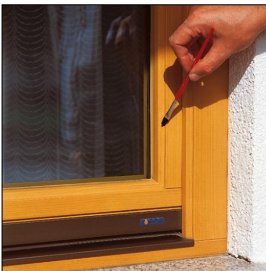
Fig. 4.1: Repair of damage
