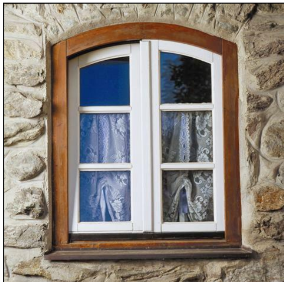
Fig. 4.2: Before renovation coating
