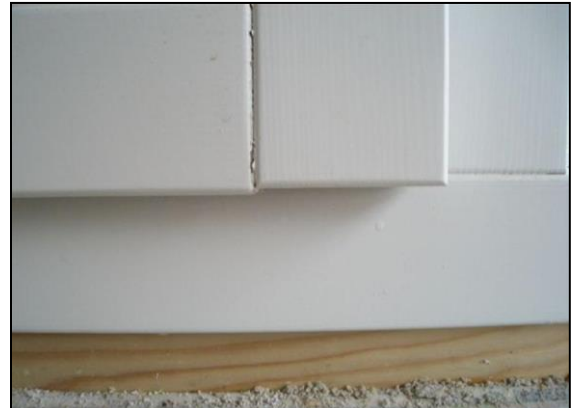
Fig. 3.3: Opened V-joint
